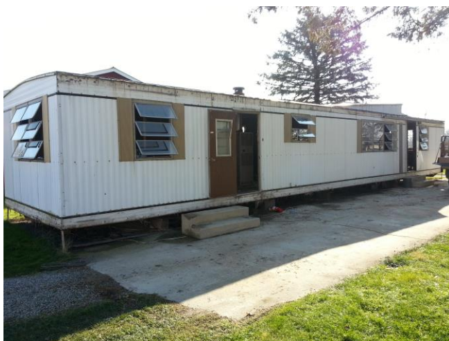
Step One- Remove awning and skirting from mobile home.
